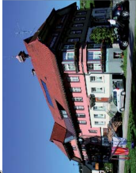
In-dachanlage Solarthermie
